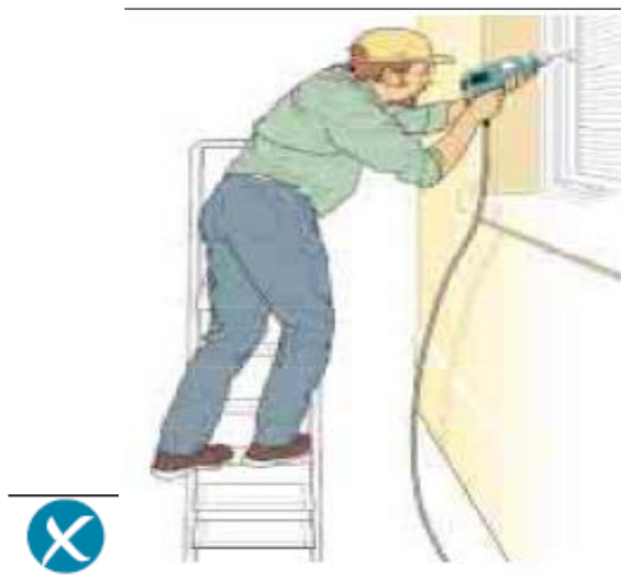
Incorrect – steps side on to work activity
