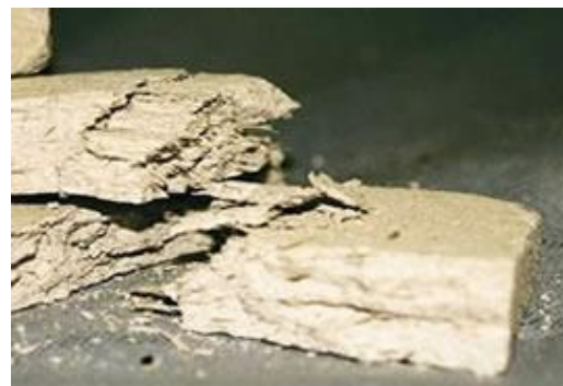
Pieces of Asbestos Insulating Board (AIB)
