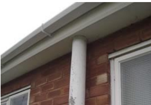
Asbestos cement drainage pipe (downpipe)
