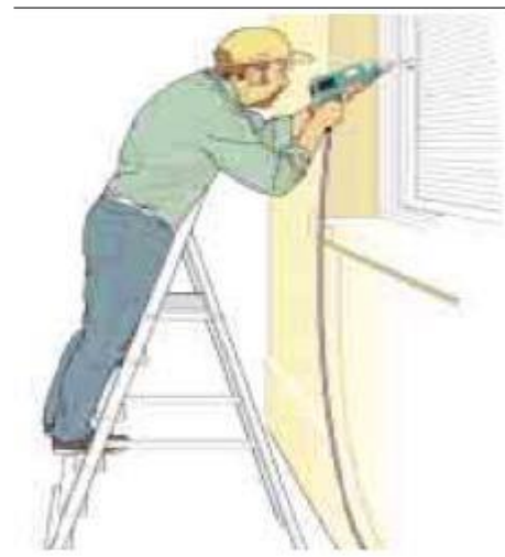
Correct – steps facing work activity
